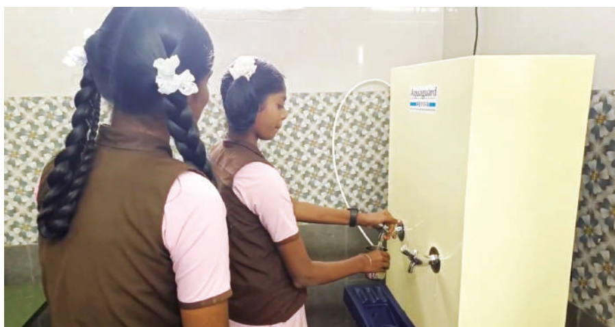
Oil and Natural Gas Corporation Ltd sponsored infrastructure development projects at Eklavya Model Residential Higher Secondary School, Kumuli (Chengalpattu).
