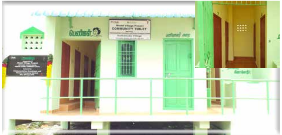
Toilet complex at Nathamedu village
