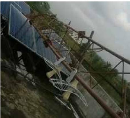
**Solar panels and communication tower destroyed by high velocity winds**
